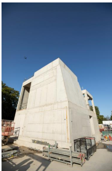
Fig.1 Head house structure complete
