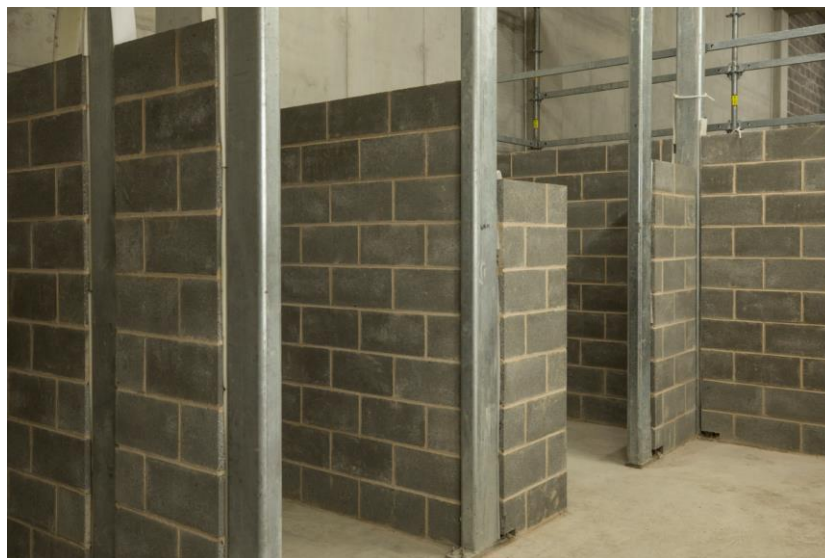
Fig. 2 Blockwork and internal rooms over 75% complete
